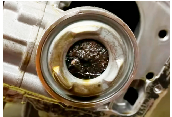
Figure 1: Oil pump intake pipes that are clogged by debris from the timing belt
